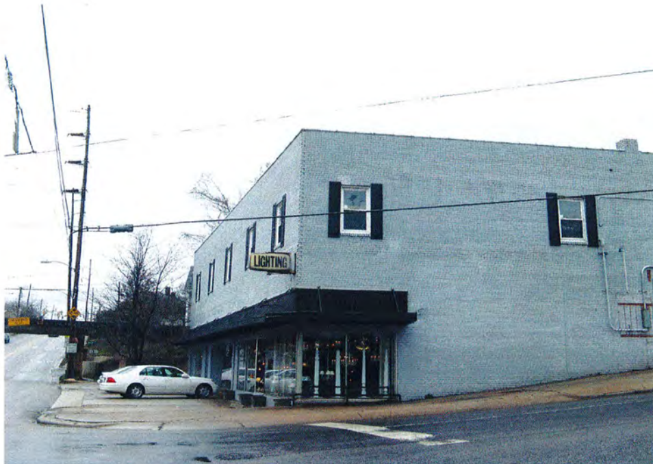
No. 7 Commercial Building, 500 West Peace Street, Looking West.
