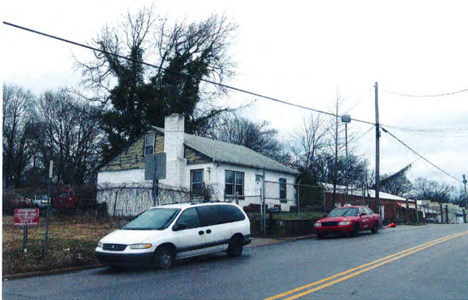
No. 9 House/Office, 713 North West Street, Looking Northwest.
