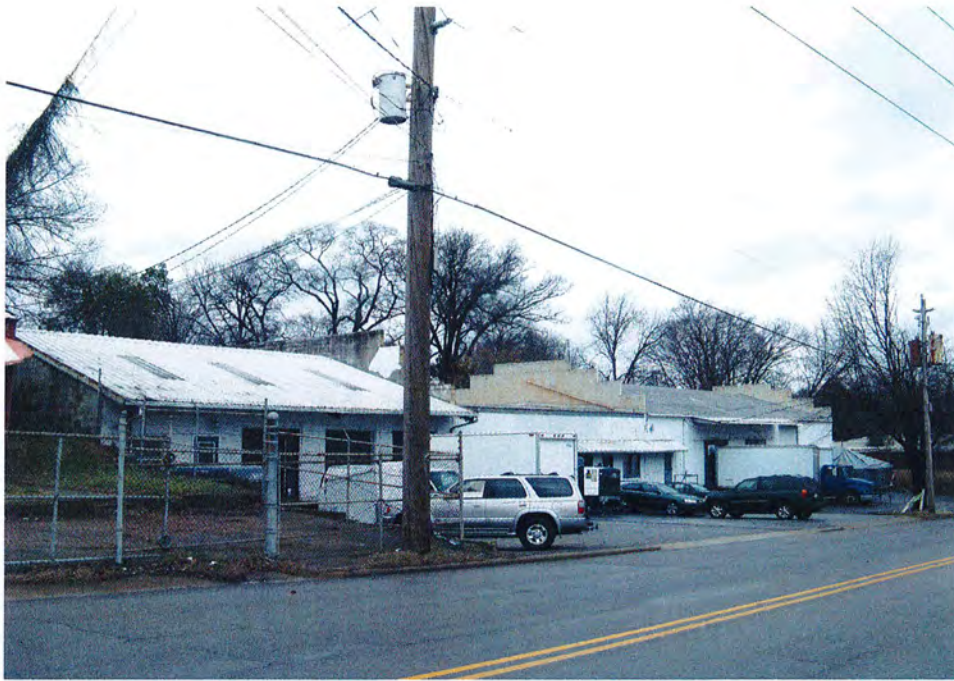
No. 12 Warehouse, 805 North West Street, Looking Northwest.
