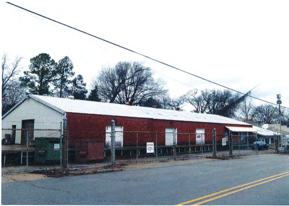
No. 10 Warehouse, 715 North West Street, Looking Northwest.
