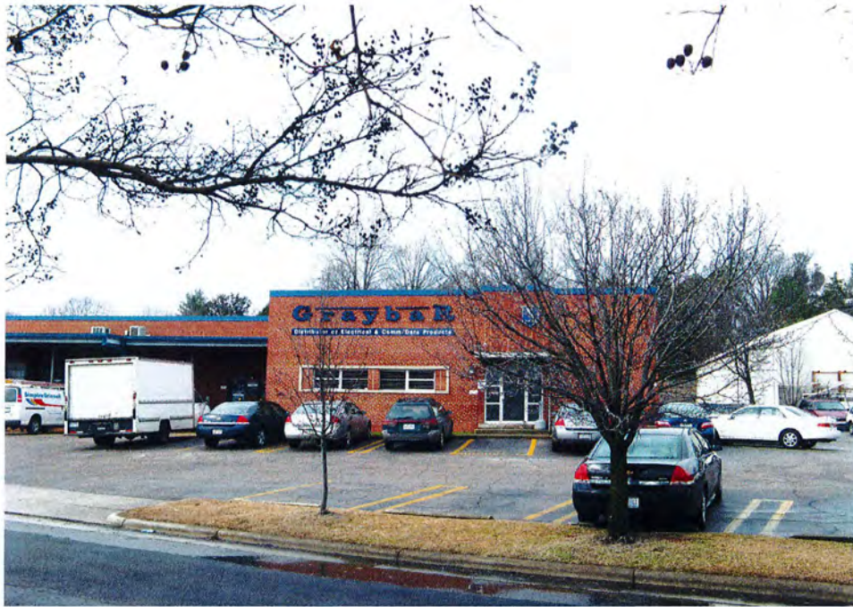
No. 14 Graybar Company Building, 1113 Capital Boulevard, Looking West.
