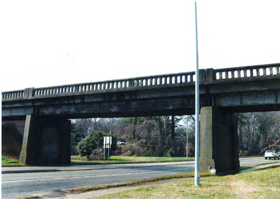
No. 4 Norfolk Southern Railway Bridges, Wade Avenue, Looking West.
