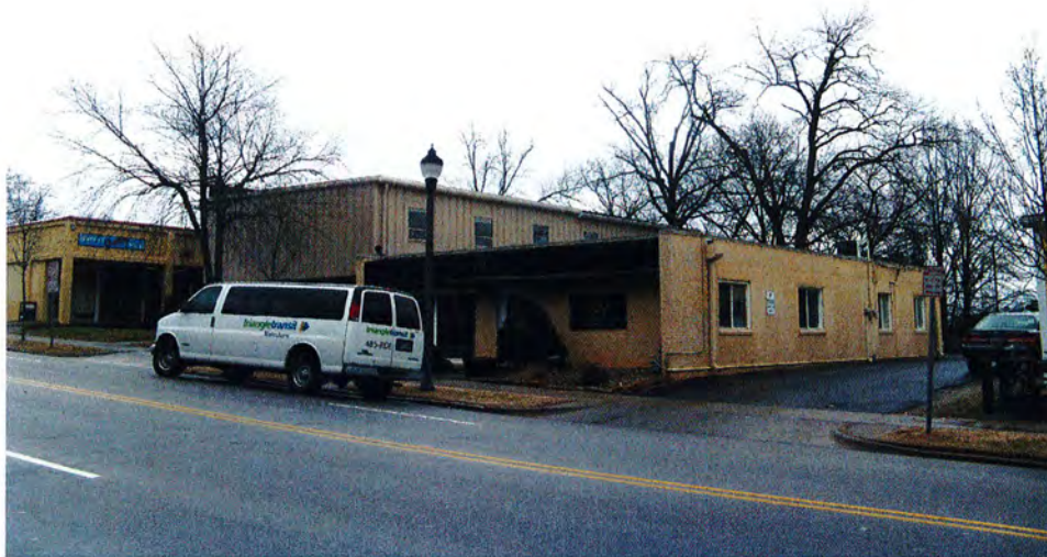
No. 6 Commercial Block, 600 Block Glenwood Avenue, 612 Glenwood Avenue.
