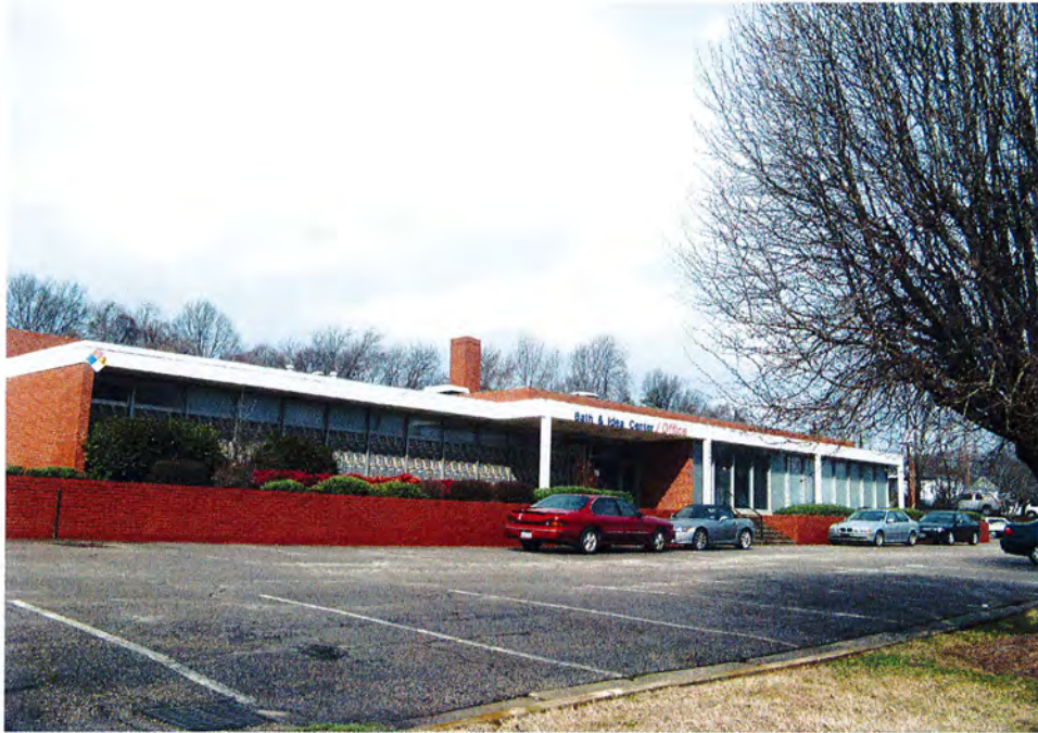
No 15 Noland Plumbing Company Building, 1117 Capital Boulevard, Looking North.
