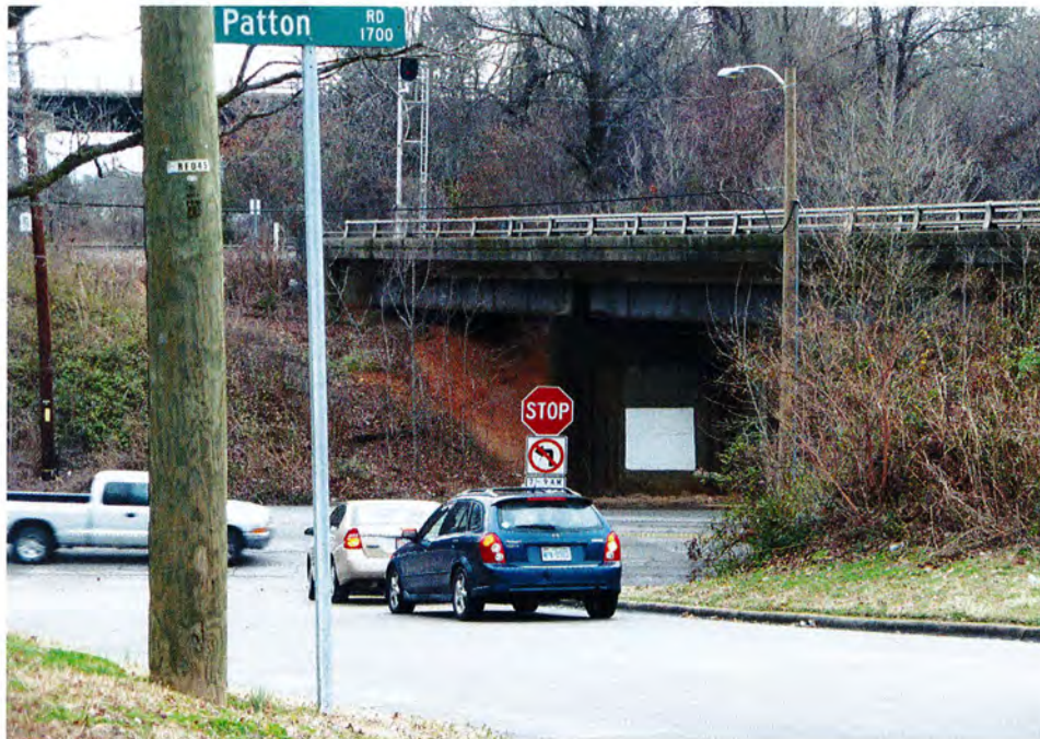
No. 28 Norfolk Southern Railway Bridge, Crossing Wake Forest Road, Looking Northeast.
