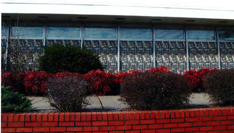
No 15 Noland Plumbing Company Building, 1117 Capital Boulevard, Façade, Looking West.
