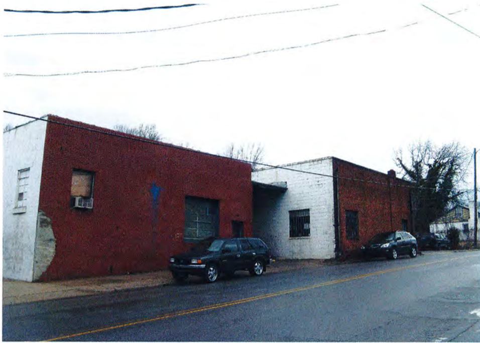
No. 8 Warehouse, 707-707 North West Street, Looking Northwest.
