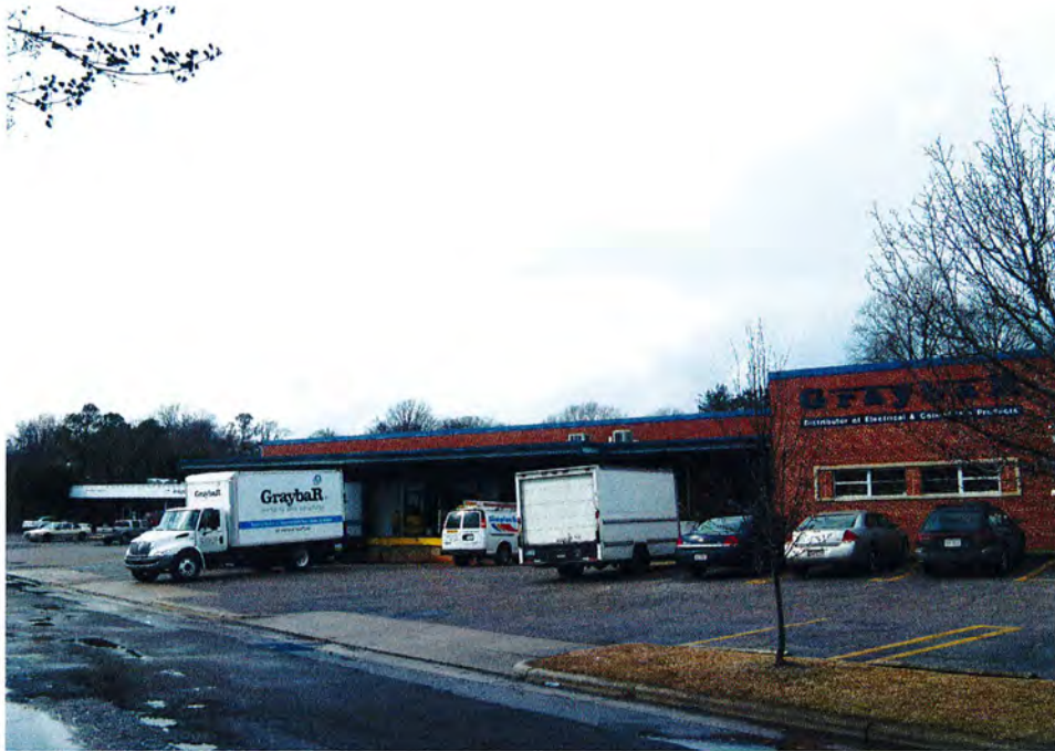
No. 14 Graybar Company Building, 1113 Capital Boulevard, Looking Southwest.
