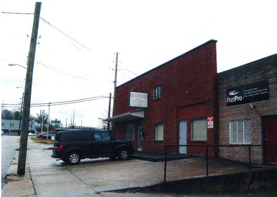
No. 3 Commercial Building, 510 North West Street, Looking North.
