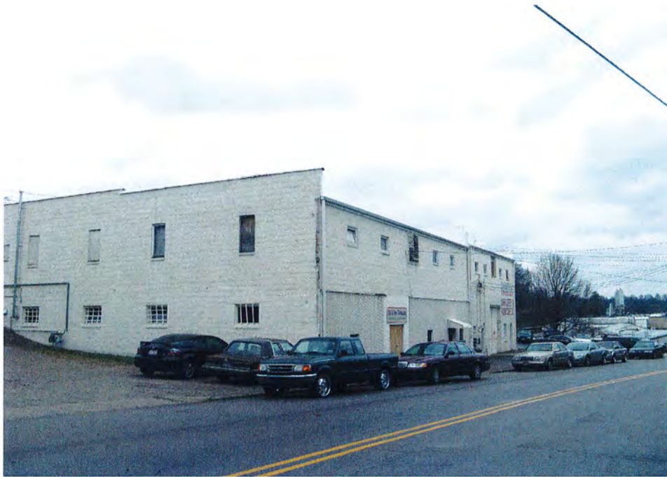
No. 13 Warehouse, 911 North West Street, Looking Northwest.
