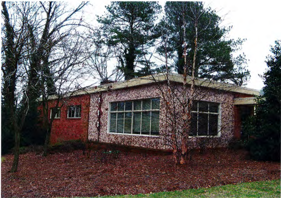
No. 32 Office Building, 333 Wade Avenue, Looking Southeast.
