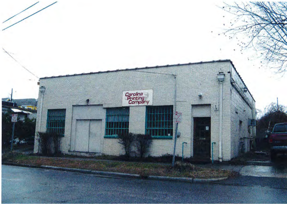
No. 5 Commercial Building, 510 West Johnson Street, Looking East.
