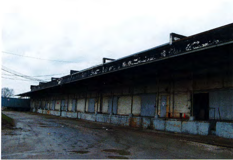
No. 30 Raleigh Bonded Warehouse, 1505 Capital Boulevard, Looking South.
