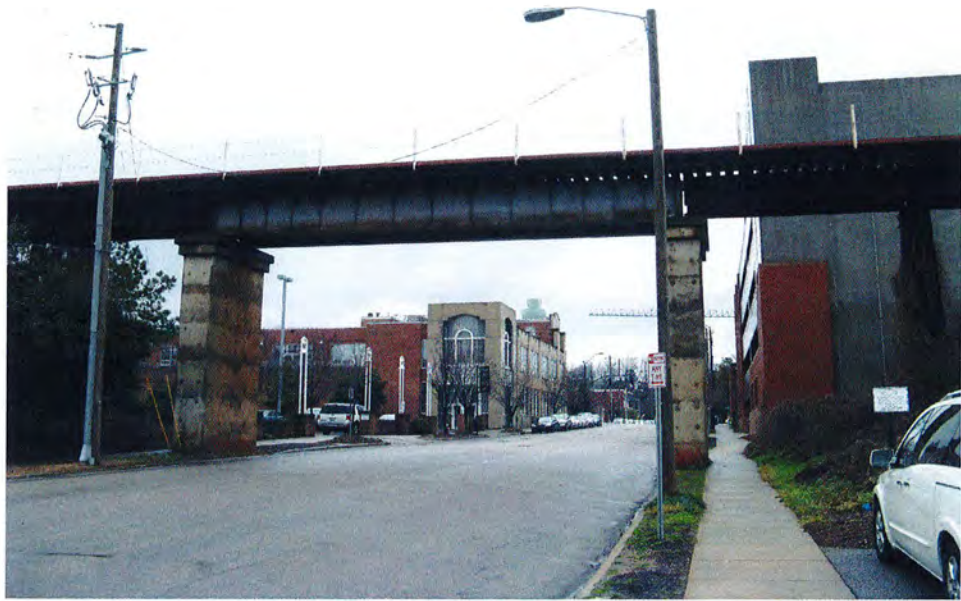
No. 4 Norfolk Southern Railway Bridges, Tucker Street, Looking West.
