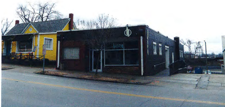
No. 6 Commercial Block, 600 Block Glenwood Avenue, 606-610 Glenwood Avenue.
