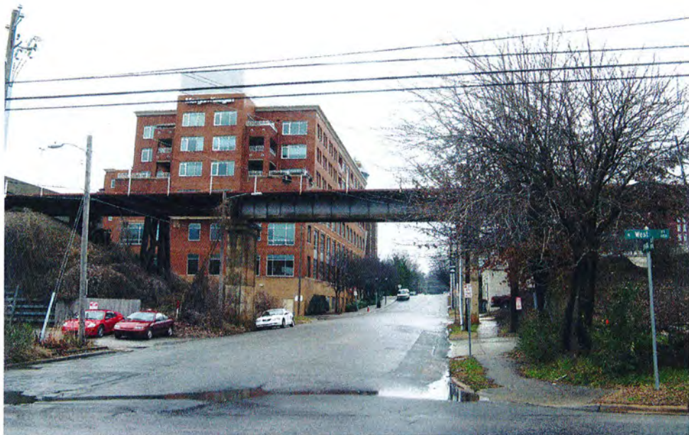
No. 4 Norfolk Southern Railway Bridges, West Johnson Street, Looking West.
