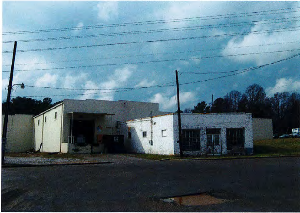
No. 19 Warehouse, 1501 Sunrise Avenue, Looking South.
