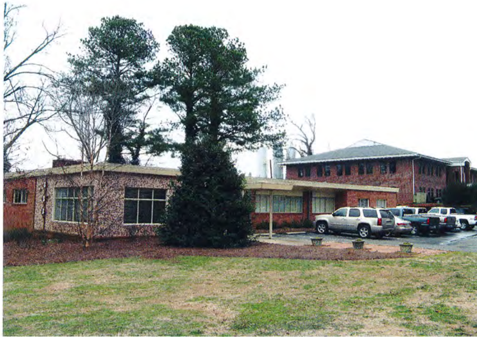
No. 32 Office Building, 333 Wade Avenue, Looking Southeast.
