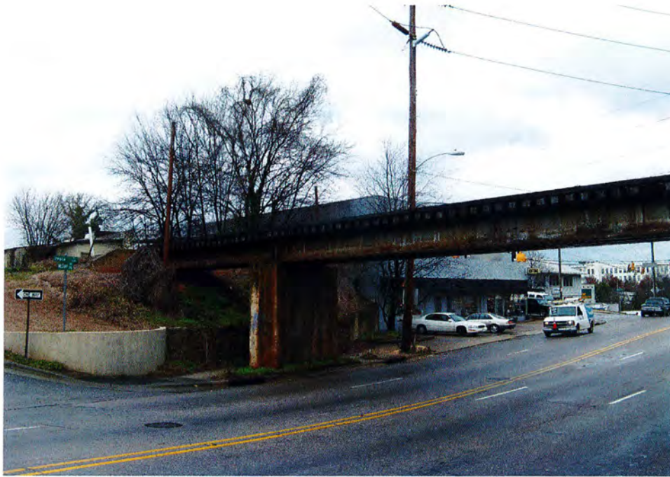
No. 4 Norfolk Southern Railway Bridges, West Peace Street, Looking East.
