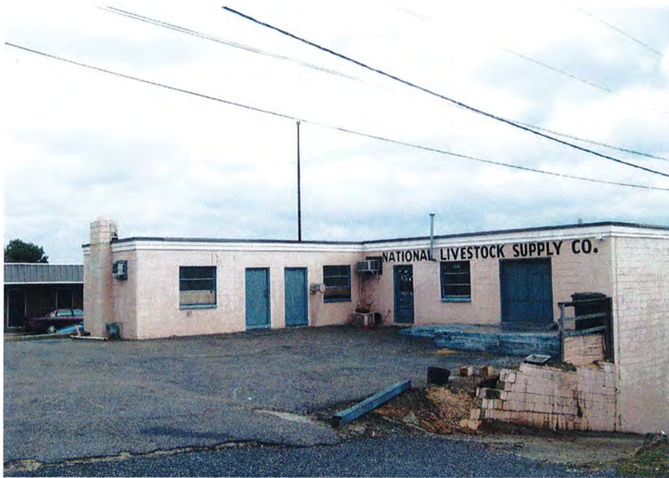
No. 11 Warehouse, 804 North West Street, Looking East.
