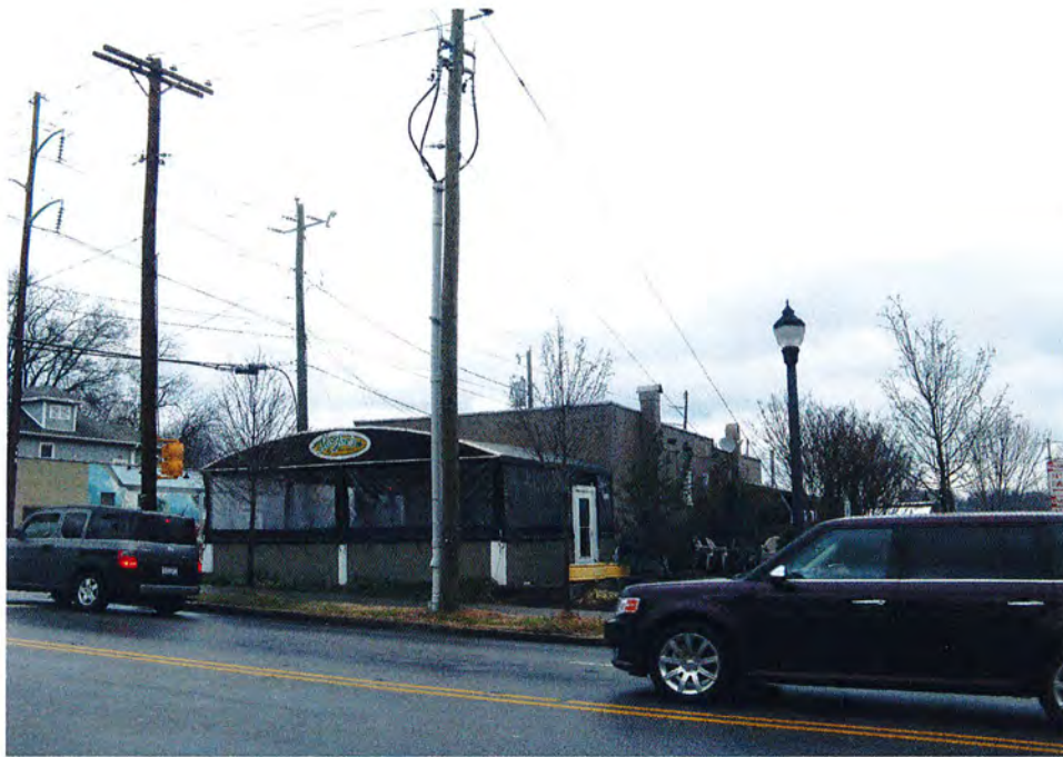
No. 6 Commercial Block, 600 Block Glenwood Avenue, 620 Glenwood Avenue.
