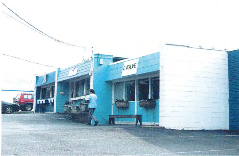
No. 17 Commercial Block, 209-215 Bickett Boulevard, Looking North.
